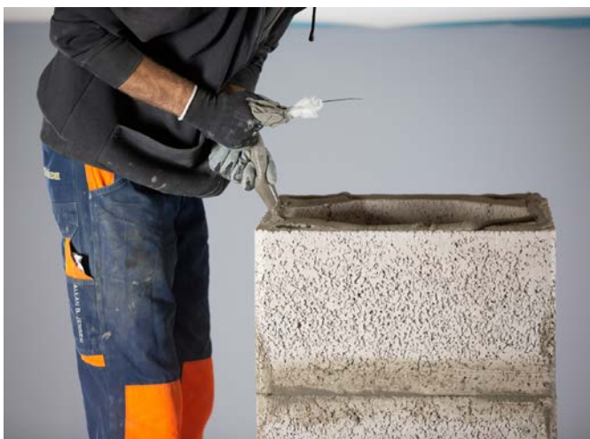
Glue on the next two chimney blocks.
