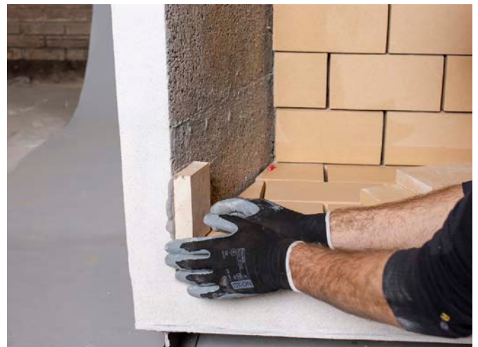
Once the bottom and rear firebricks are in place, fasten the side bricks in position using the firebrick mortar. Use a tile spacer to keep an 8mm gap.
