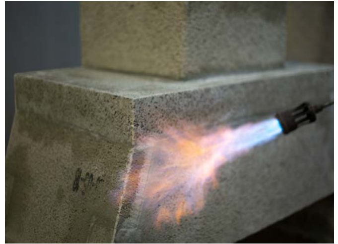
Burn off the fibres on the external surface before rendering.
