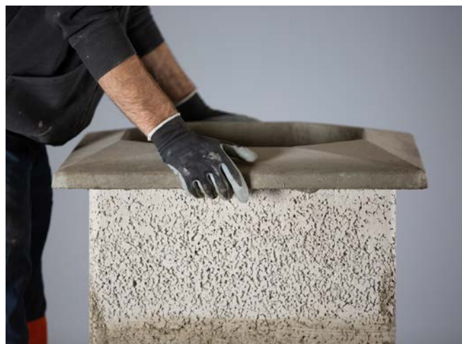
Glue on the capping.
