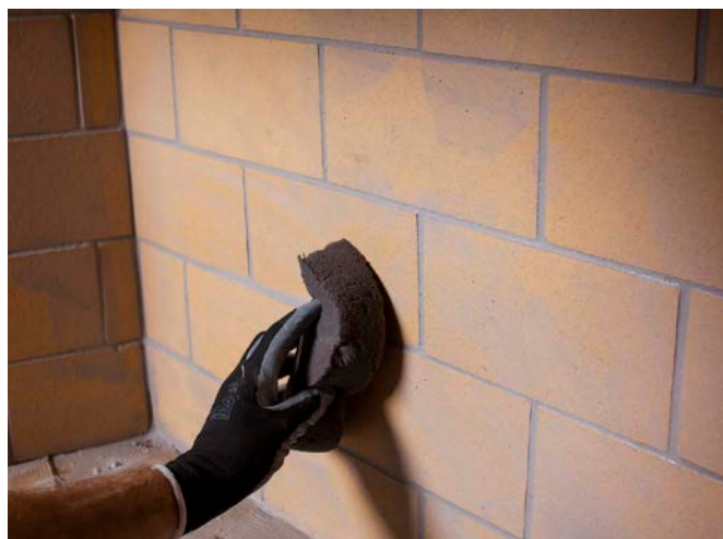
Clean off excess mortar.
