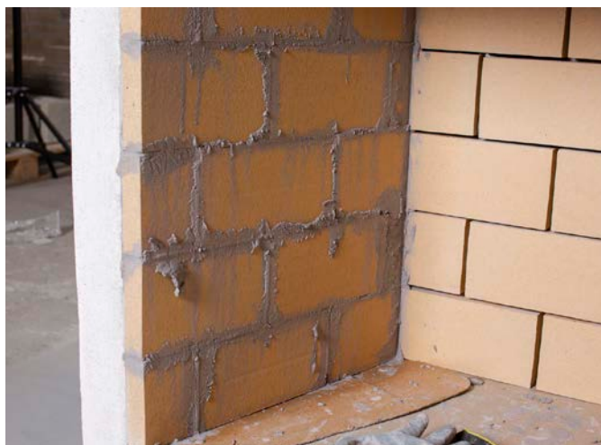
Use the mortar mix to point up the joints between the firebricks once they are all in position.
