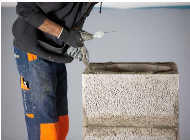
Glue on the next two chimney blocks.
