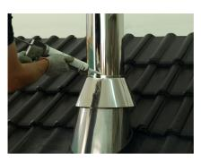
Apply a silicone mastic to the joint between the collar and the chimney.
