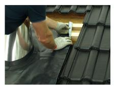
Fold the side edge of the membrane up to form drainage barrier.
