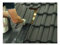
12. Cut roof tiles to appropriate shape to fit around the cone of the chimney.
