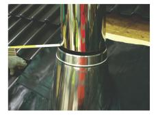
3. Center the flashing by measuring distance from the chimney to the perimeter on the edge of the cone.
