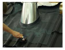
6. Use the roller to press the Wakaflex firmly to the tiles to ensure a tight connection.
