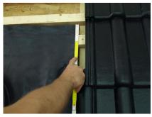
8. The batten should be nailed 5 cm below the upper edge of the Wakaflex membrane.
