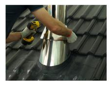
15. Install a storm collar and tighten the screw to fit tightly to the chimney pipe.
