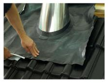
4. Tear off the foil on bottom edge and press the flashing slightly to the tiles to retain the flashing's position.
