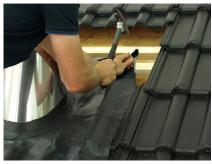
11. Lay the Wakaflex membrane on to the batten and fix in place with nails on the right hand side, left hand side and in the centre.
