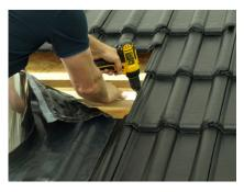
Cut to length and nail down the batten over rafters located to the left and right side of the chimney
