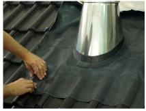
Mold on Wakaflex flashing on to the tiles to bottom, left and right side of the channel (from hip to water channel).
