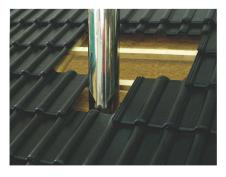
First step: chimney pipe is installed though the roof. Leave a line of roof tiles above the chimney uncovered.
