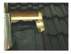
Fold the membrane upwards to form a gutter to prevent water penetration into the roof structure.
