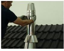
17. Install terminal and secure it with locking band.
