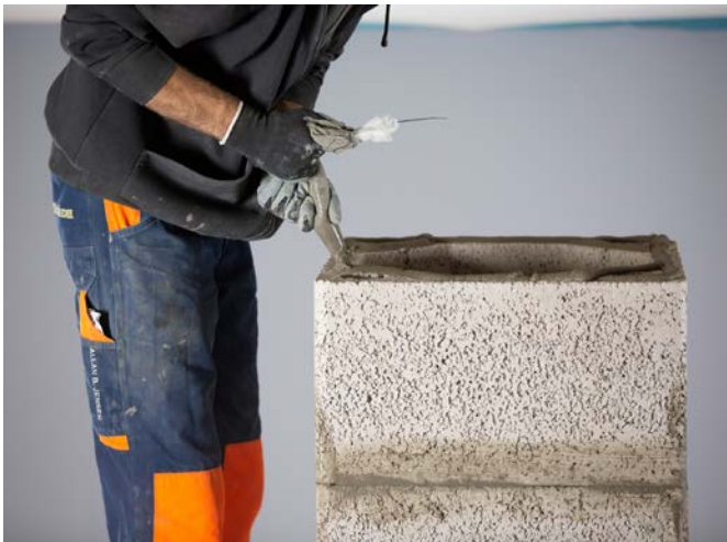
Glue on the next two chimney blocks.
