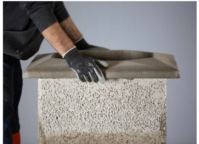
Glue on the capping.
