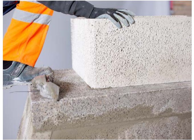
Press the first chimney block into place, checking it is in the correct position above the hole in the top plate.
