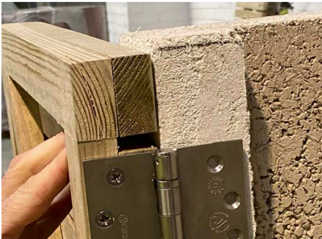
Align the hinge to the logstore, ensuring the door is below the top of the logstore (a 5mm gap is fine).
