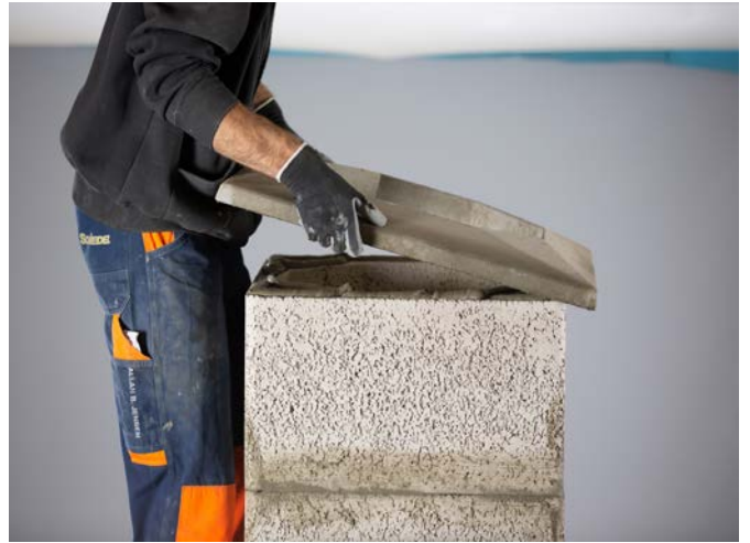
Position the capping over the glue and central.
