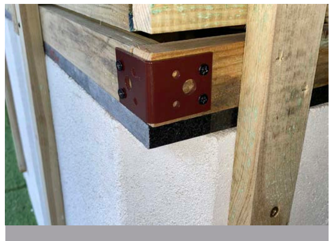
Attach the bottom metal bracket to the side and back panels.
