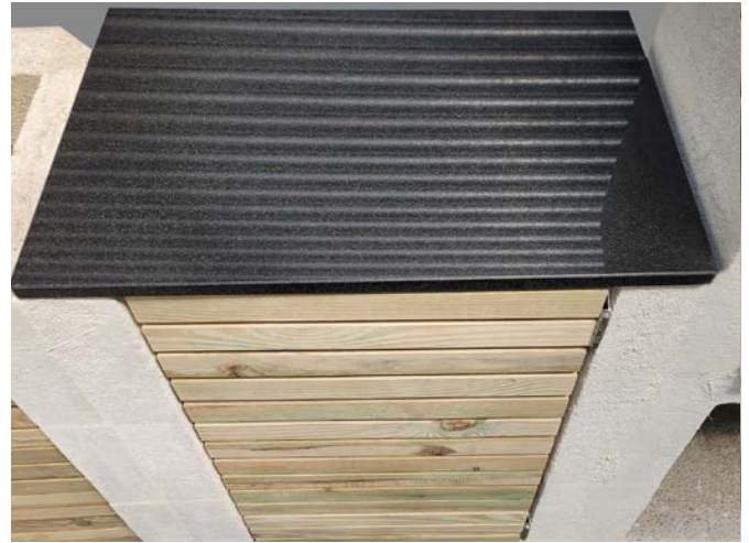
Ensure that the granite is level.
