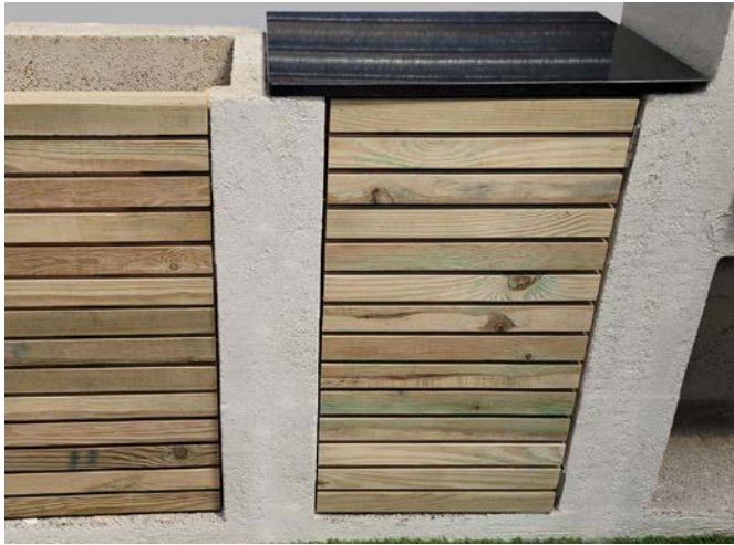
Lay the granite surface on a bed of lip glue.
