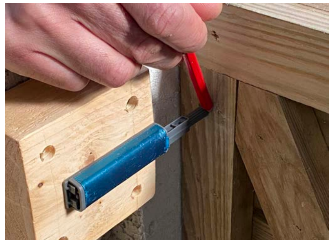
Mark with a pencil the end of the magnetic latch on the door.
