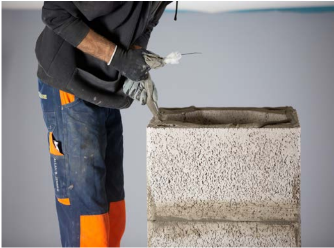
Apply lip glue to the top of the final chimney block.
