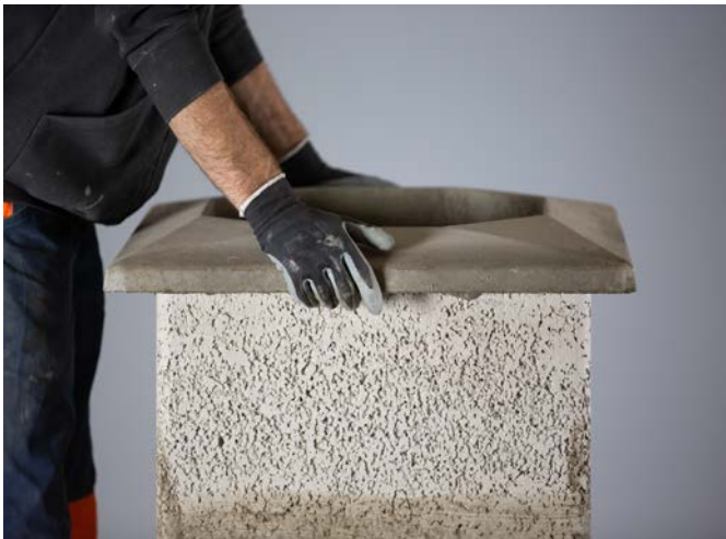
Push and adjust in to place.
