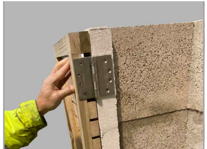
Secure the hinge to the pumice logstore with the screws provided.
