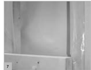
7 Install the wooden surround for Ignis-Protect into the studwork.
