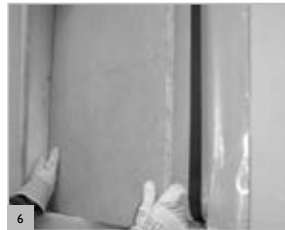
6 Remove wood fibre board, thermal insulation etc. from the assembly opening.
